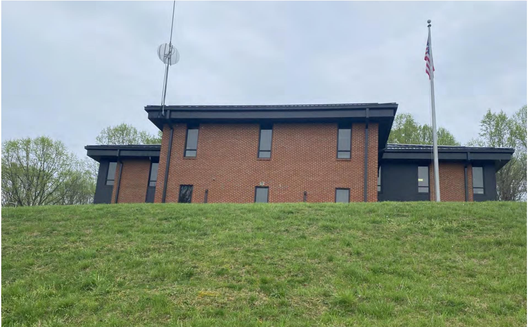
4. Site Photo - Looking South
