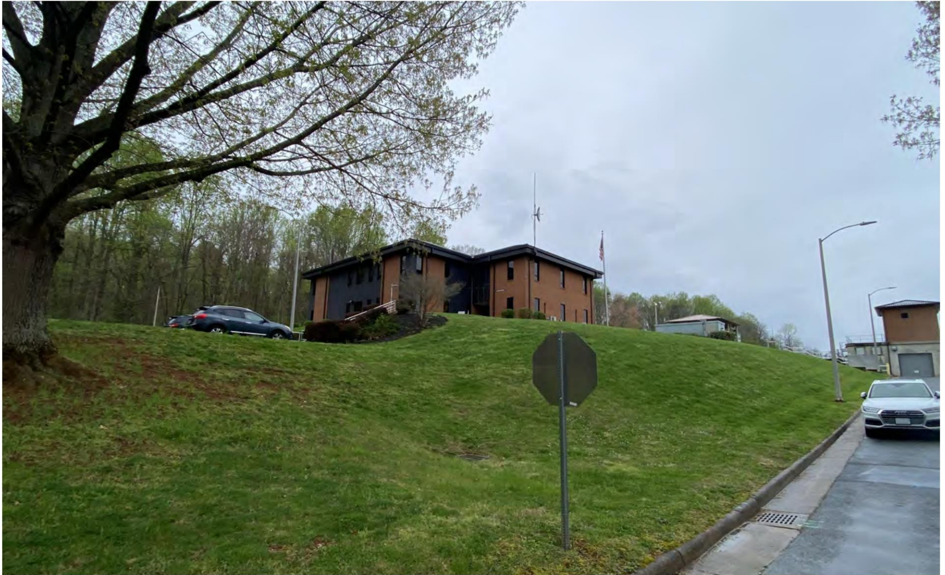
6. Site Photo, Looking Southwest
